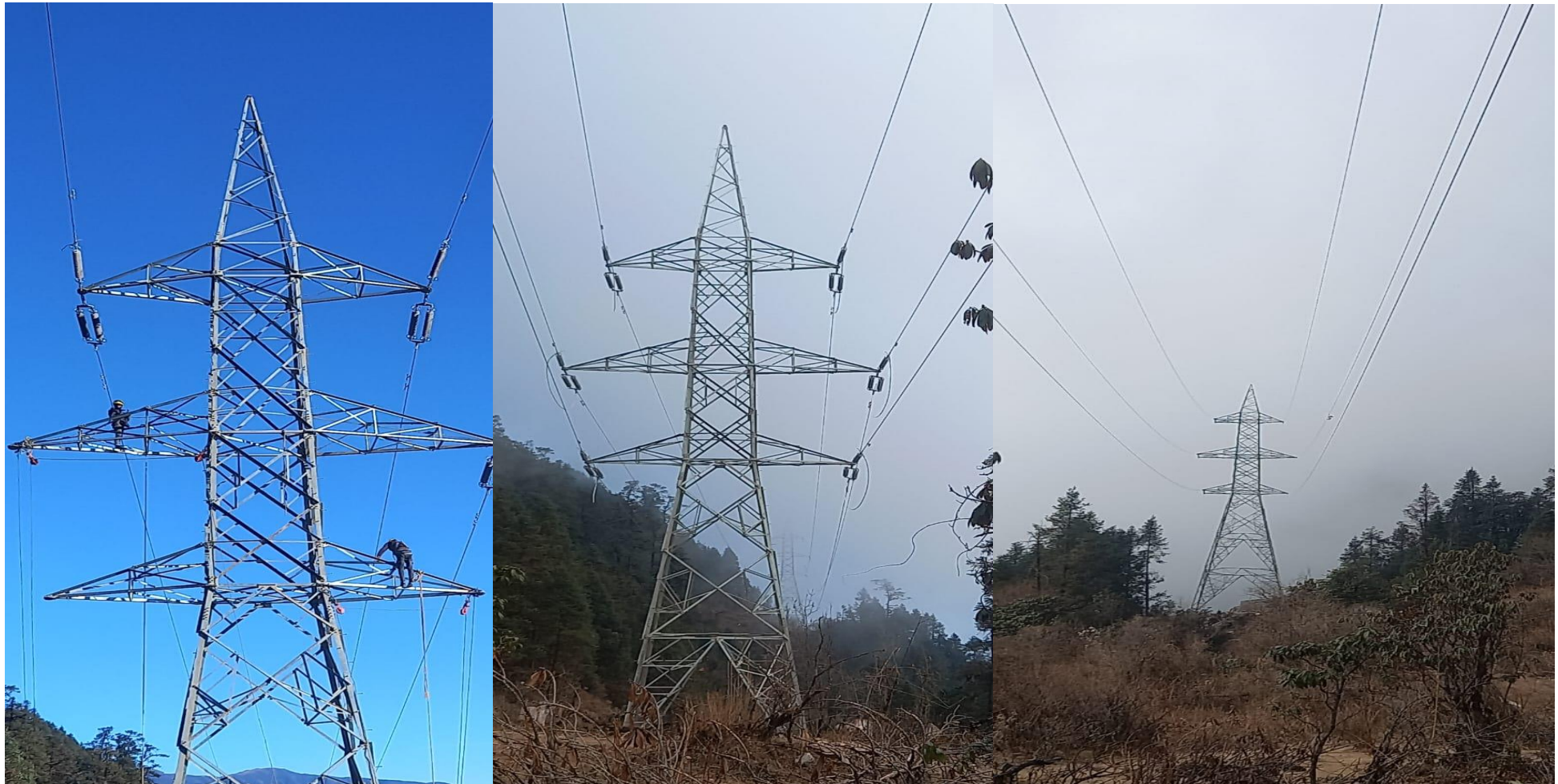
Tower Erection and Stringing Works
