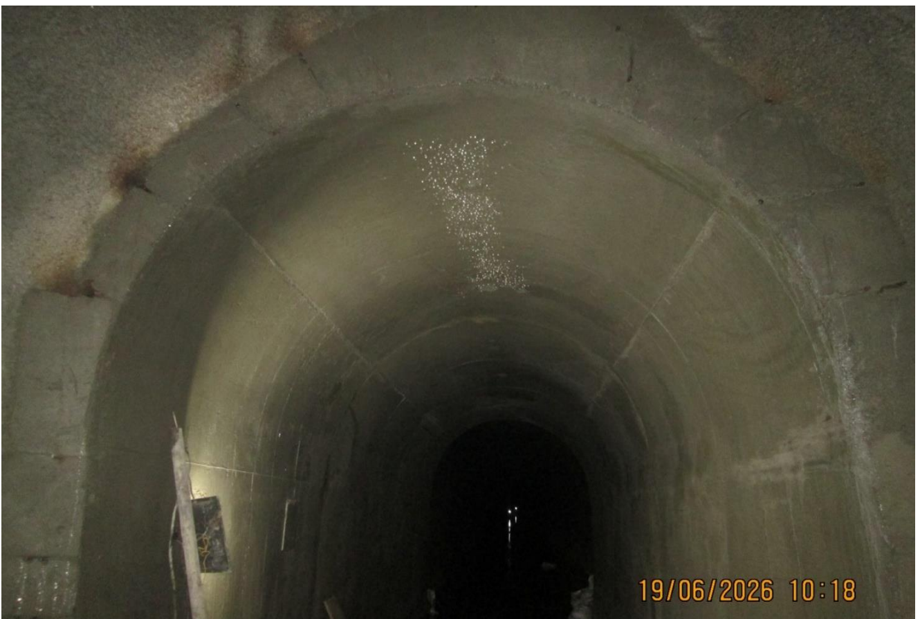
Full Concrete Lining Inside Tunnel
