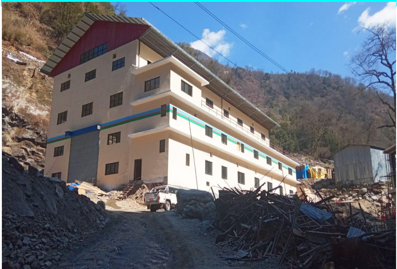
Work Progress in Powerhouse
