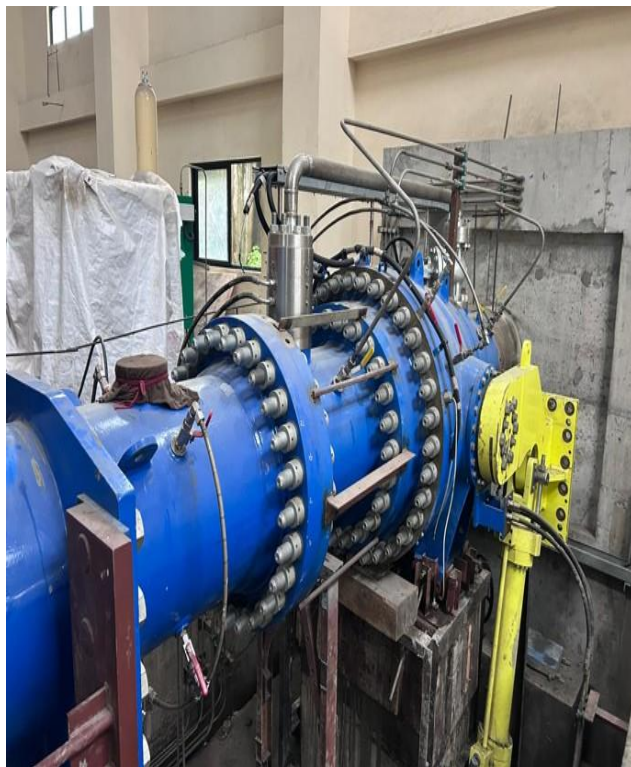
Complete erection of MIV
