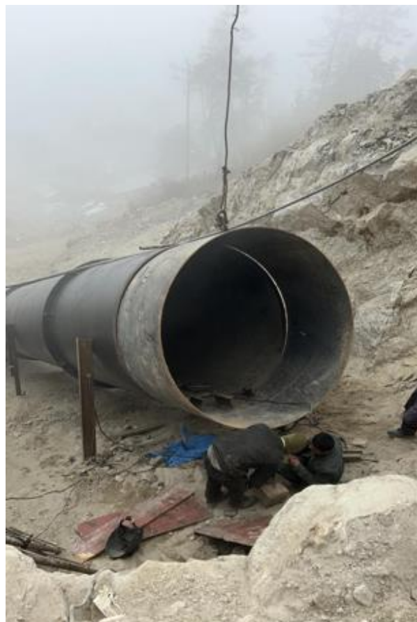
Pipe welding work at AB1 section
