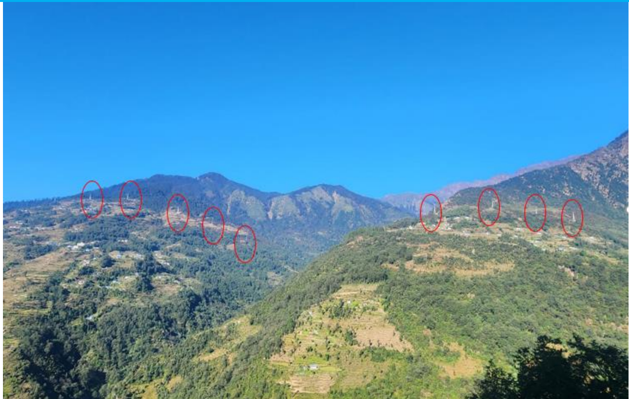
NLHP Transmission Line Towers
