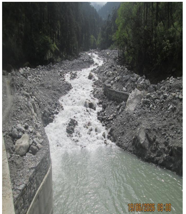
Upstream River Channelization at Likhu Intake
