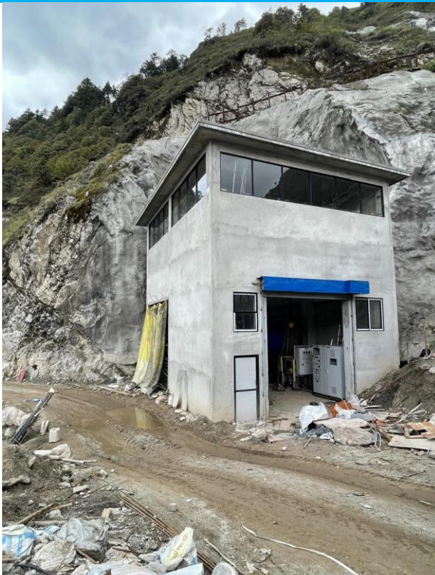
Valve House at Outlet
