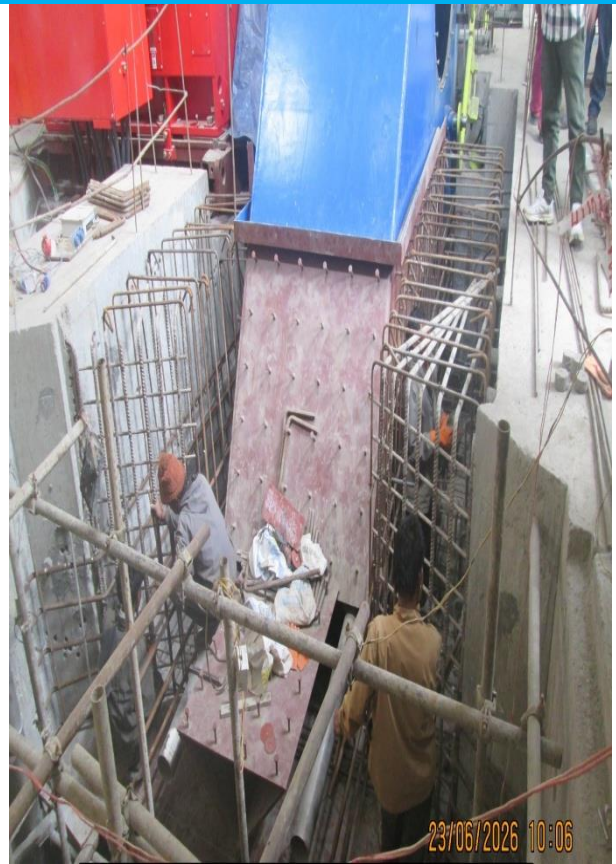
Rebar work for 3 rd Stage Concrete of Turbine
