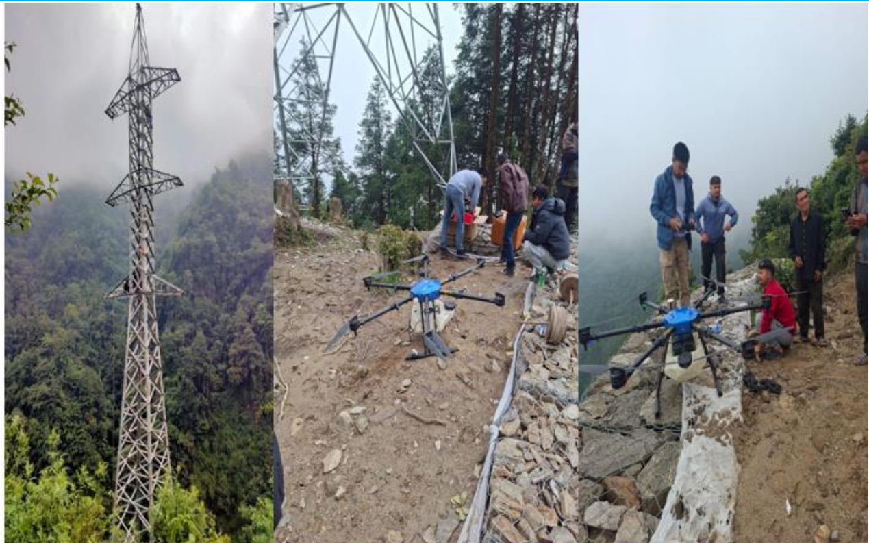
Tower Erection and Stringing Works using Drone
