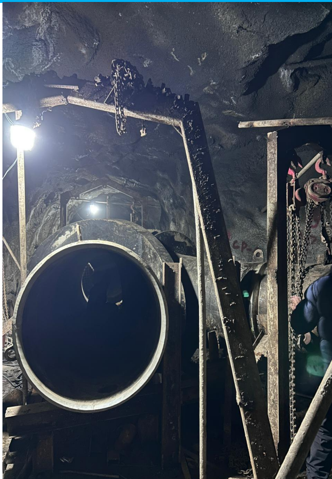
Penstock Erection at Bifurcation
