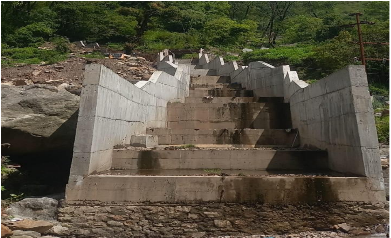
Kholi near Powerhouse
