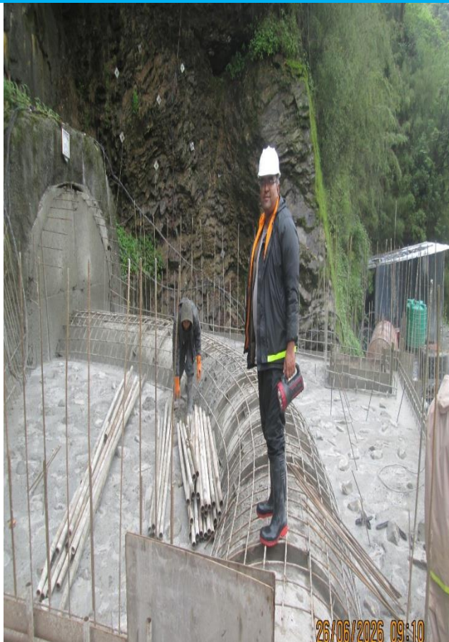
Anchor Block AB9 – Final Concrete Casting
