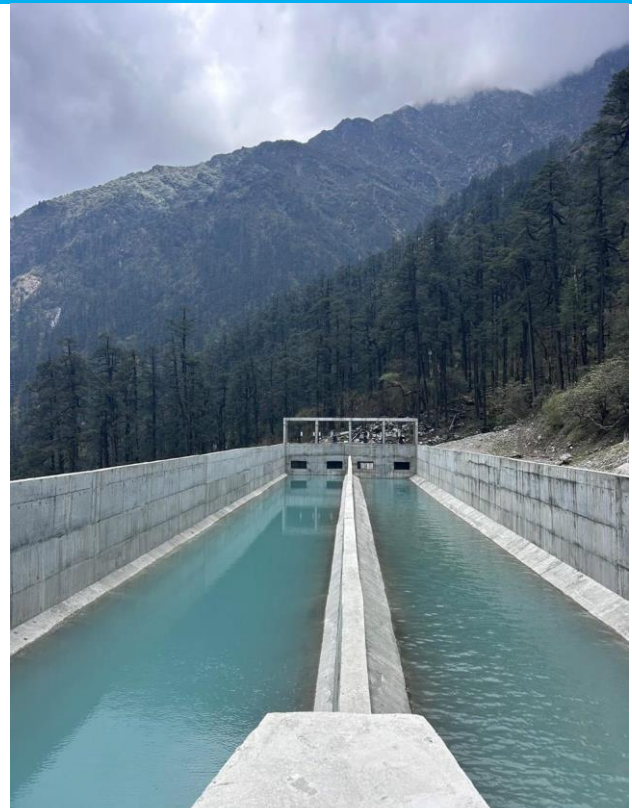
Settling Basin Testing Likhu HW
