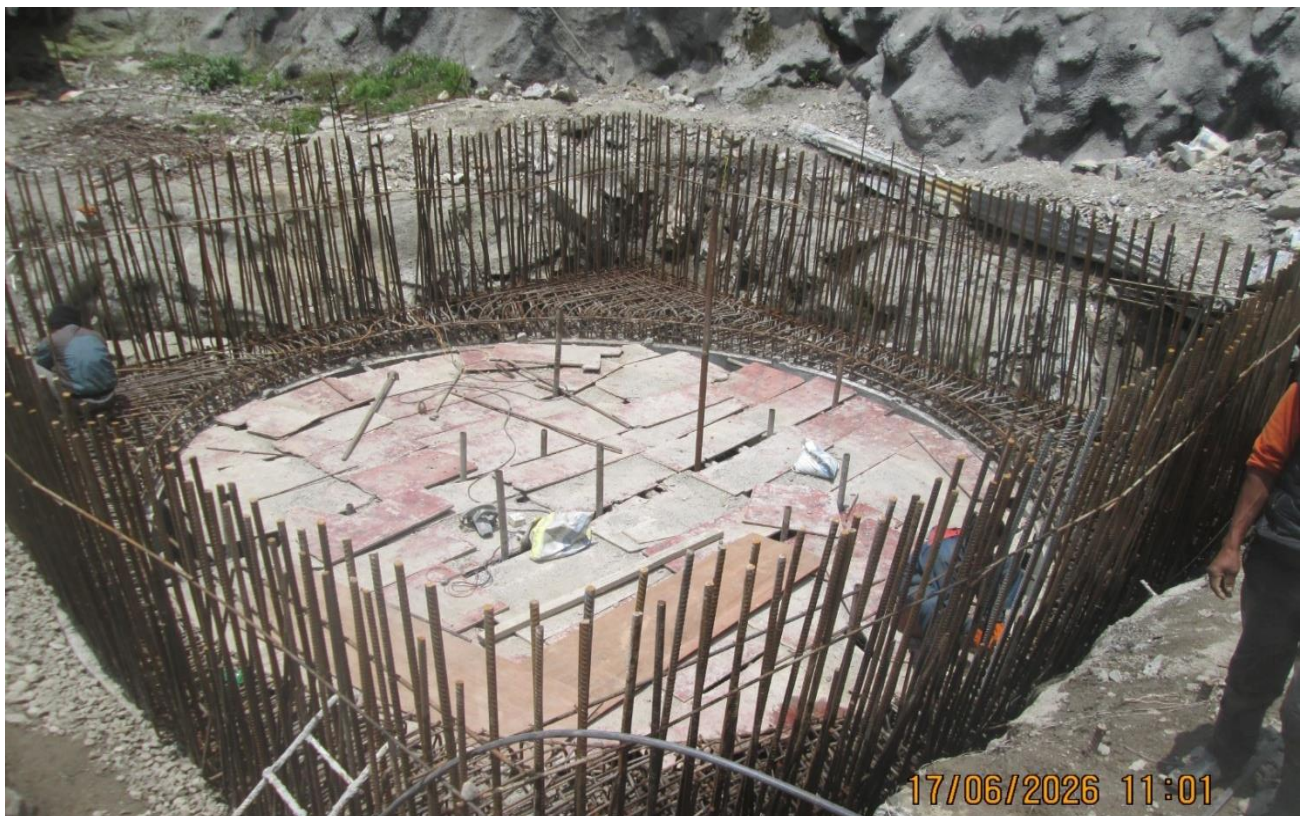
Surge Shaft Dome Reinforcement Work
