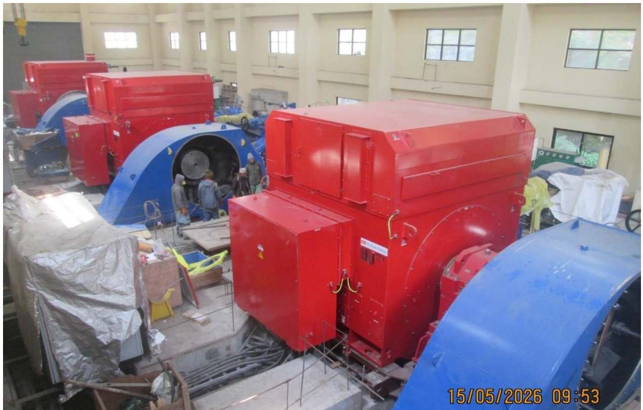
Installation of third Turbine Housing
