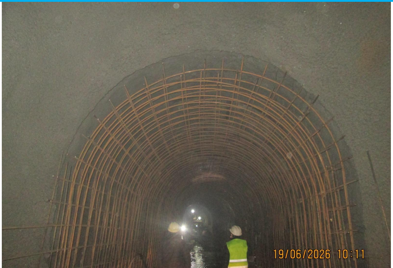
Headrace Tunnel (HRT) Reinforcement Work
