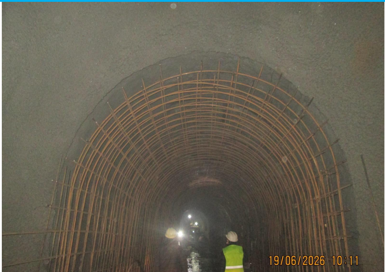
Headrace Tunnel (HRT) Reinforcement Work
