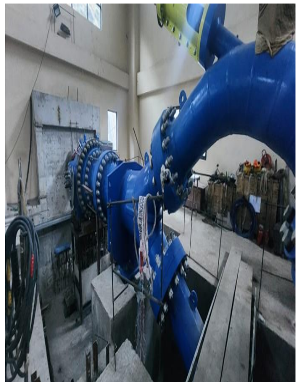
Complete erection of Nozzle
