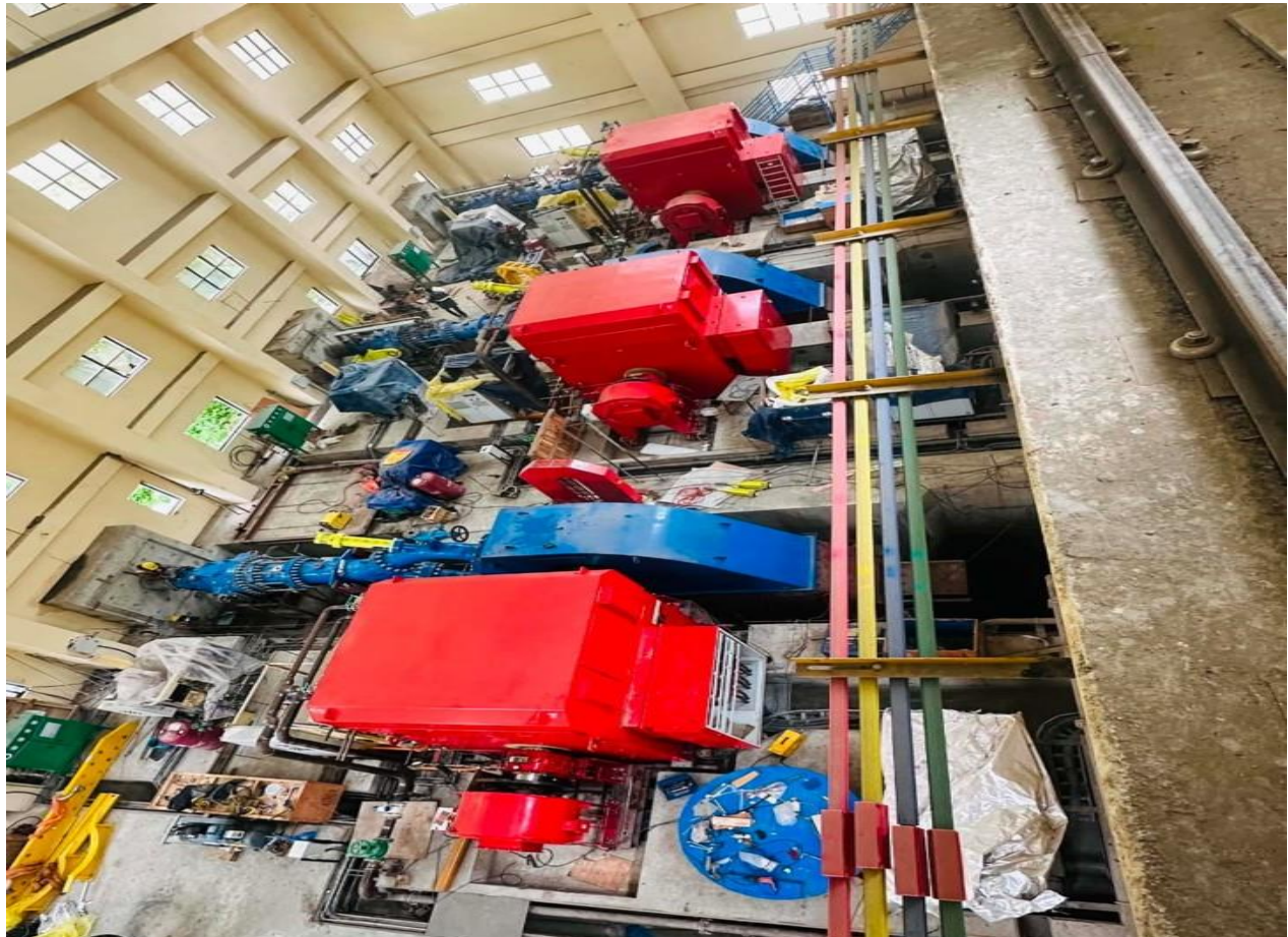
All unit Assembly completed
