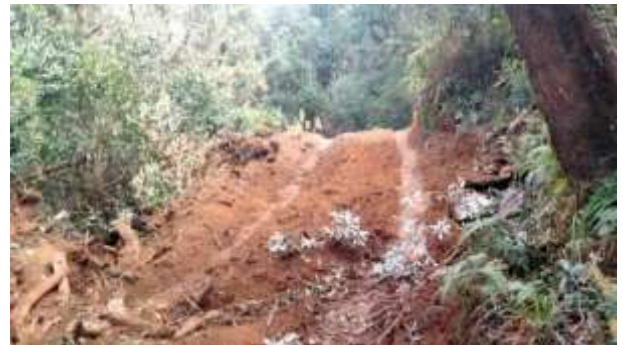
Figure: Excavation of Access road in tower area 22/2
