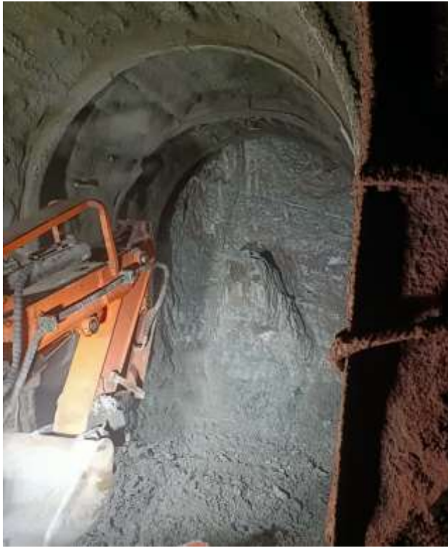
Figure: Adit Junction
