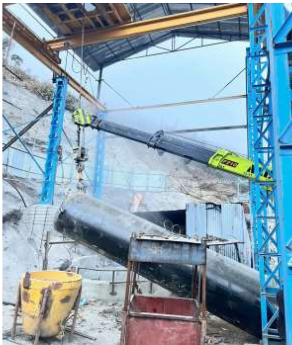
Figure showing Load Test at Vertical Shaft
