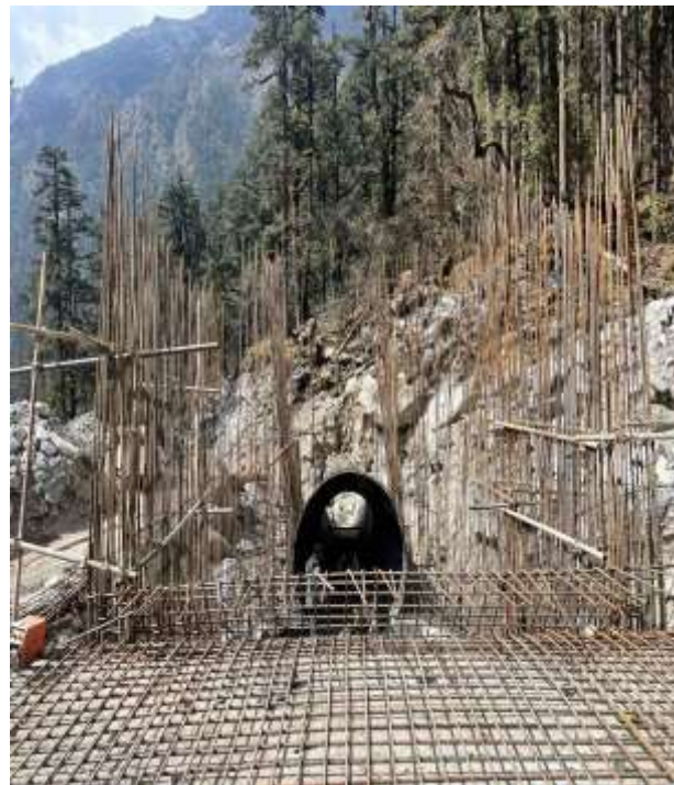
Figure: Pipe erection and Anchor Block Works
