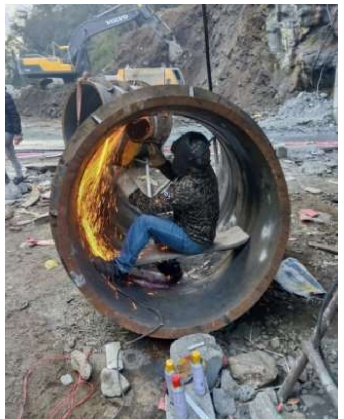
Figure: Grinding inside VS2
