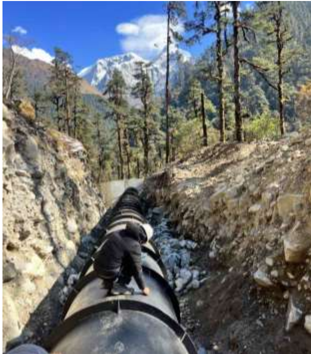
Figure: Pipe erection Works at Likhu Pipe Alignment
