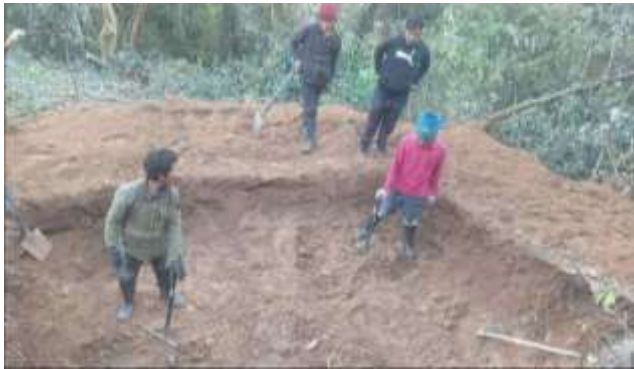
Figure: Excavation in Pit in Tower 6/2
