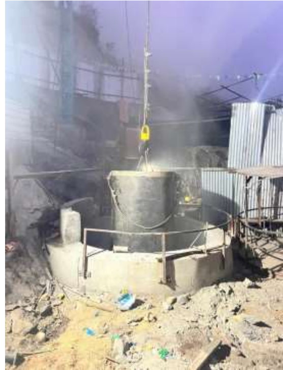
Figure: PCC work at Penstock Tunnel
