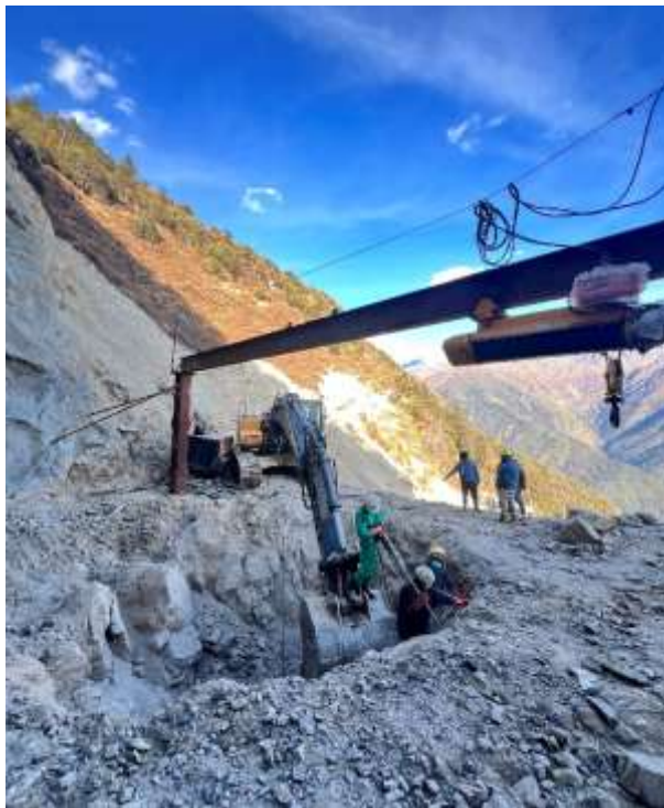
Figure: Surge Shaft Drilling
