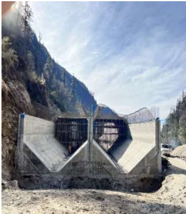
Figure: Nupche Settling Basin superstructure
