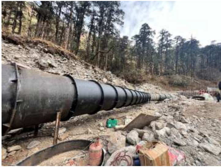
Figure: Placing of penstock pipe in alignment
