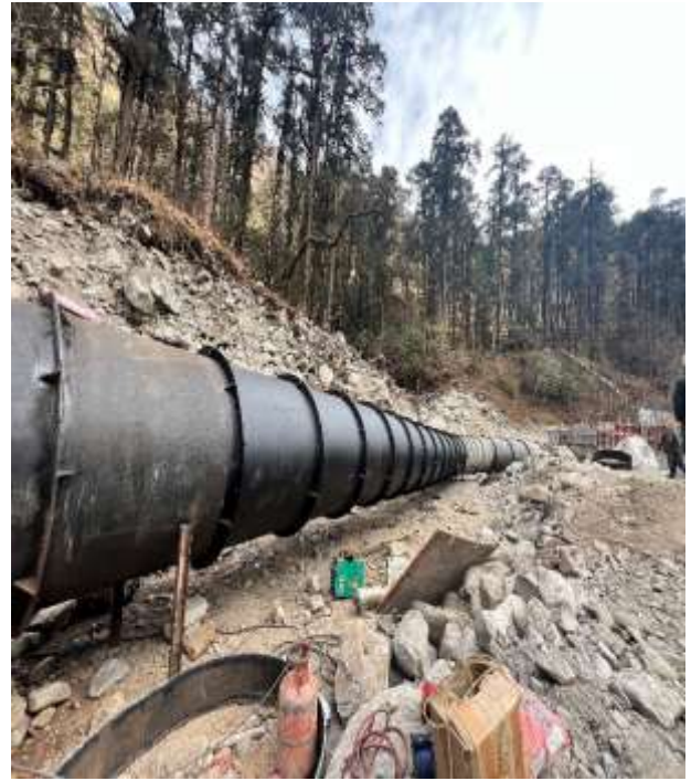
Figure: Pipe erection Works at Likhu Pipe Alignment
