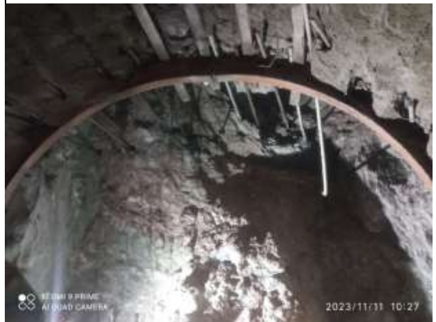
Figure: Rib Section in Adit Tunnel
