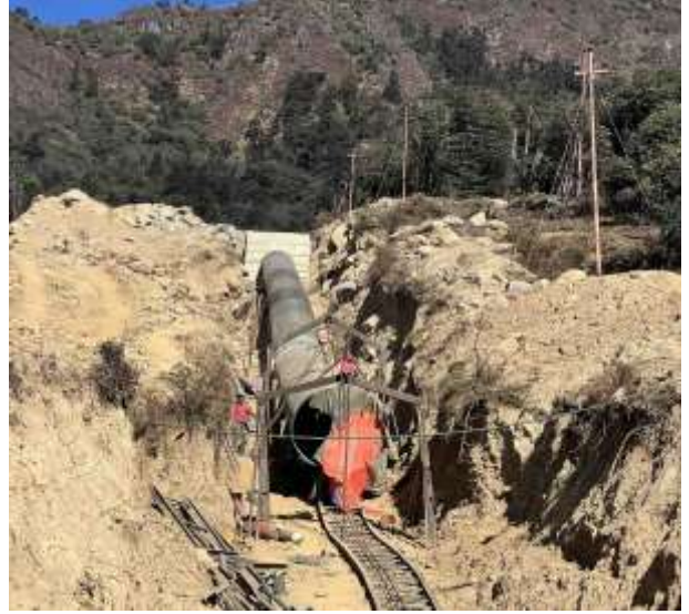
Figure: Erection of penstock pipe in alignment
