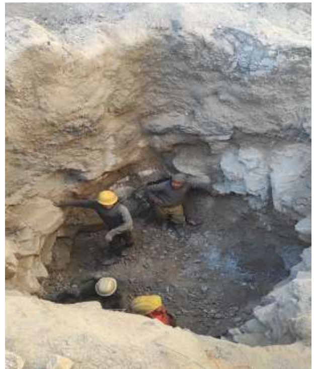
Figure: Mucking Work
