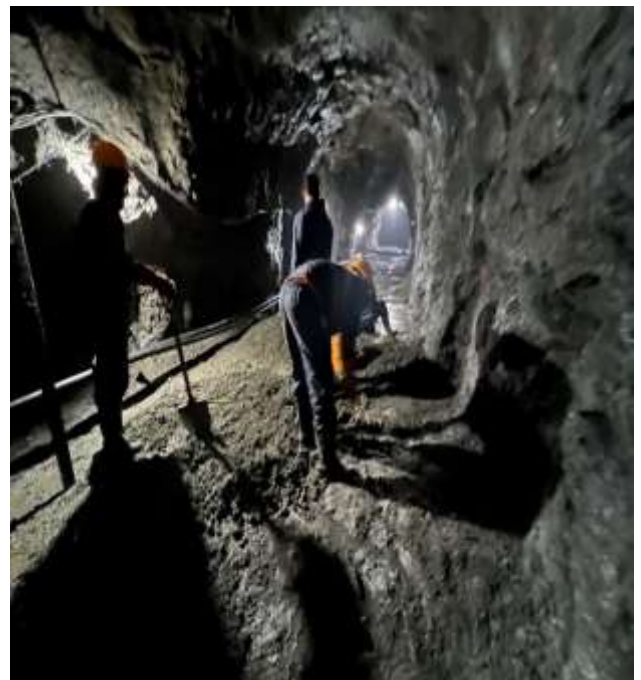
Figure: PCC work at Penstock Tunnel
