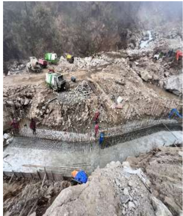
Figure: Nupche Flood Wall base concrete
