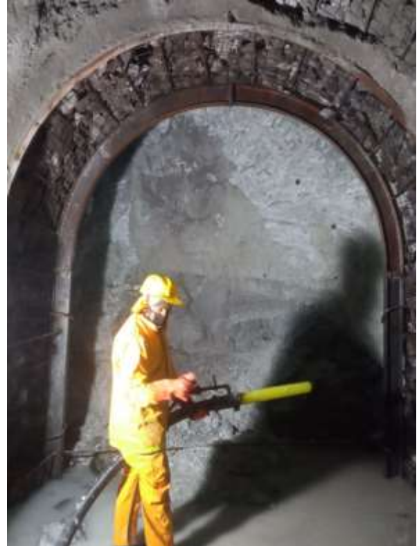
Figure: Rib Section in Adit Tunnel
