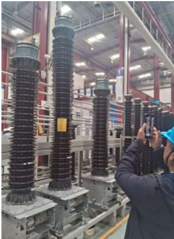
Figure: Inspection of CTs
