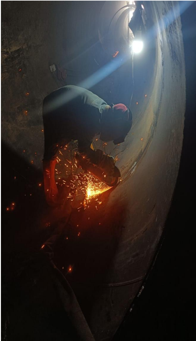
Penstock Erection Work
