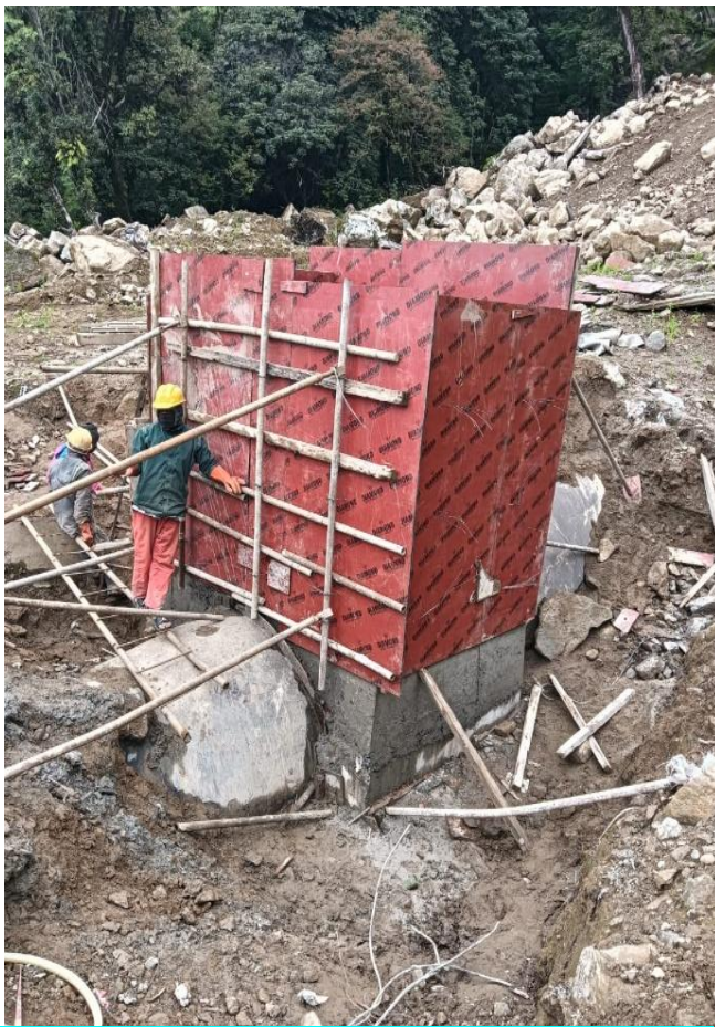
Concreting Works at Anchor Block
