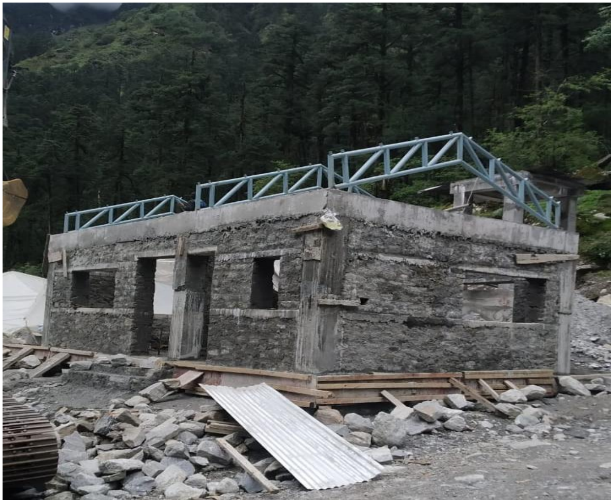
Control Building at Likhu Headworks
