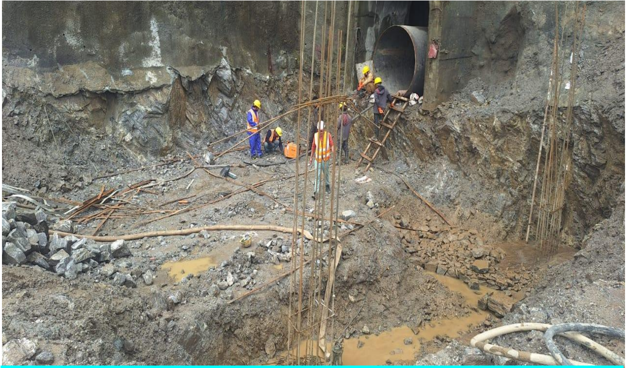
Rebar Works for Foundation at Valve House
