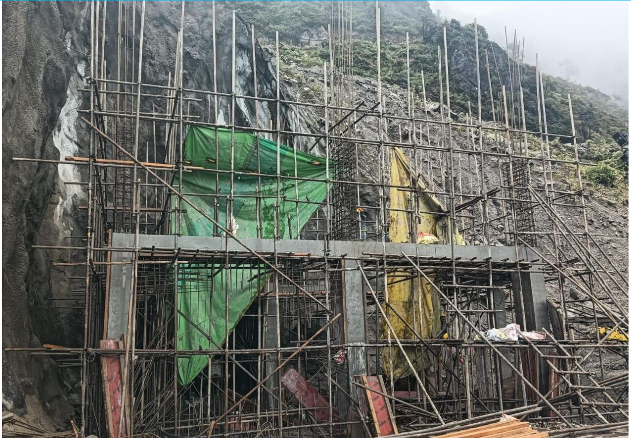
Structural Works for Valve House at Outlet
