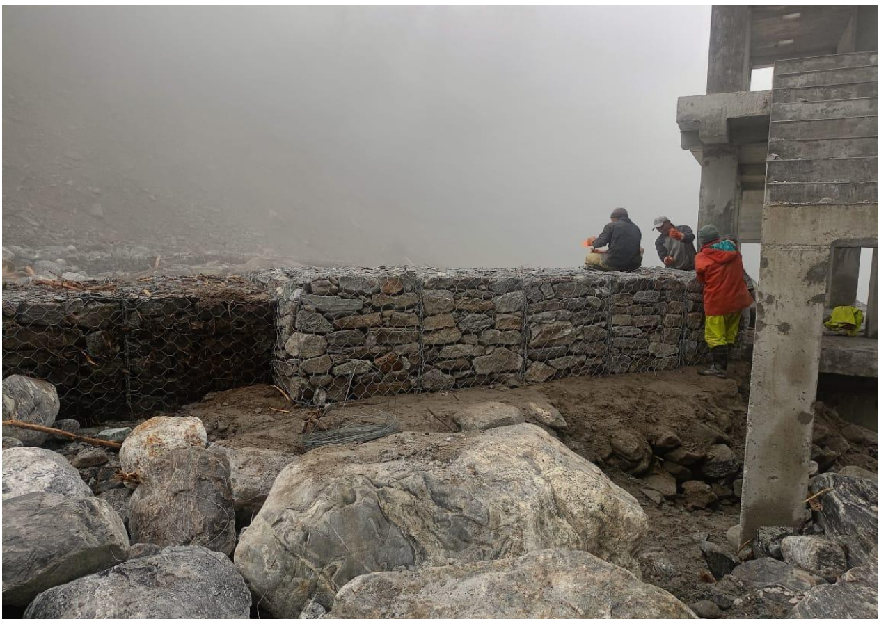
Gabion wall protection work along the river channel
