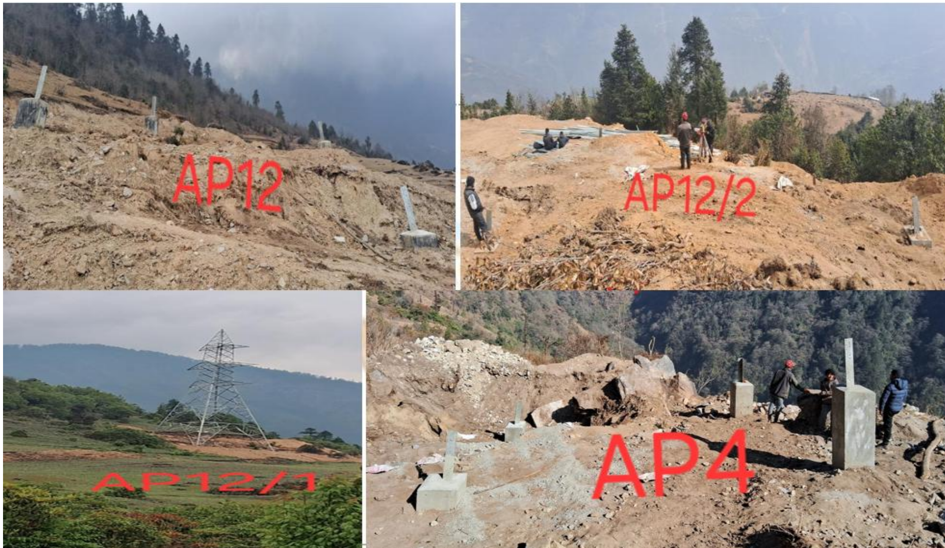
Status of NLHP Tower Foundation and Erection Works.
