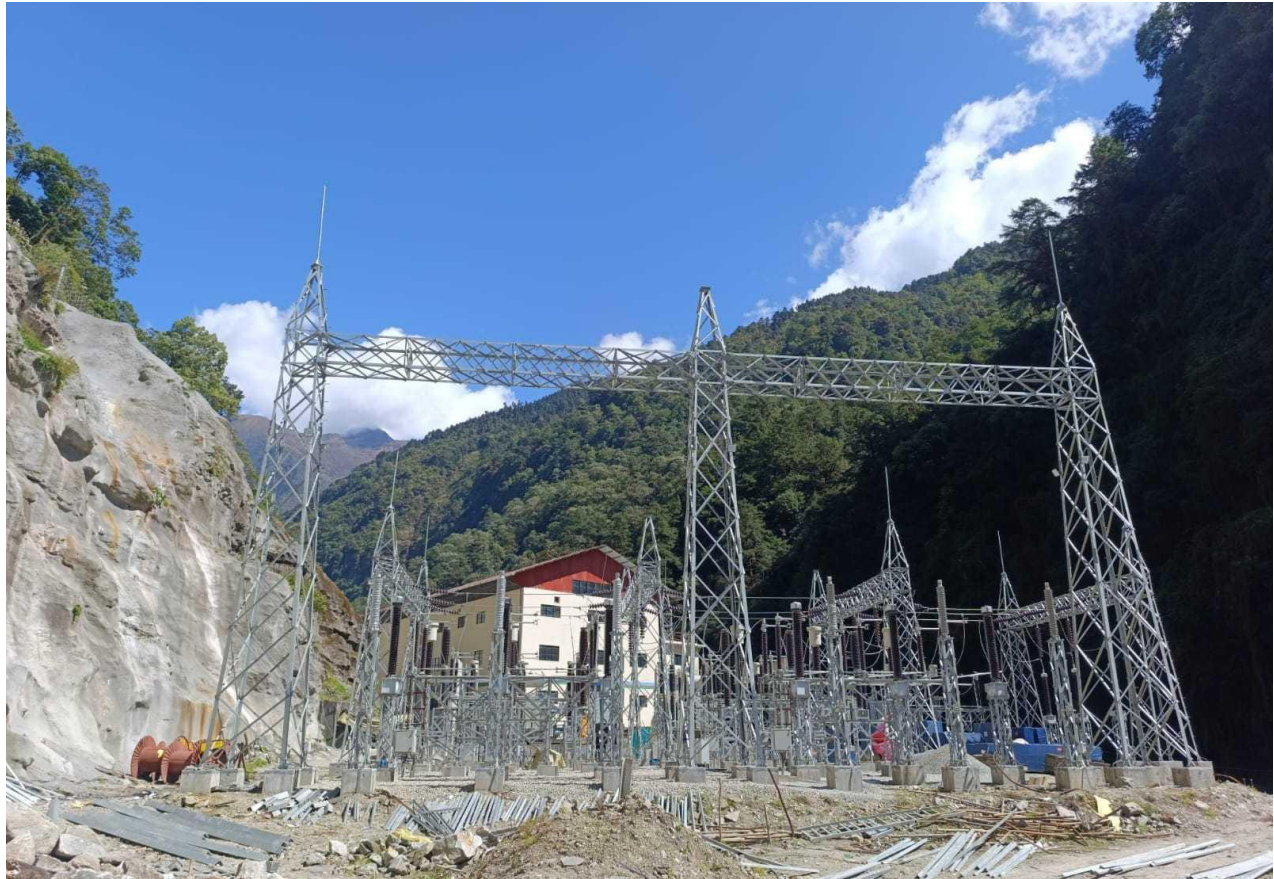
Work Progress in Switchyard
