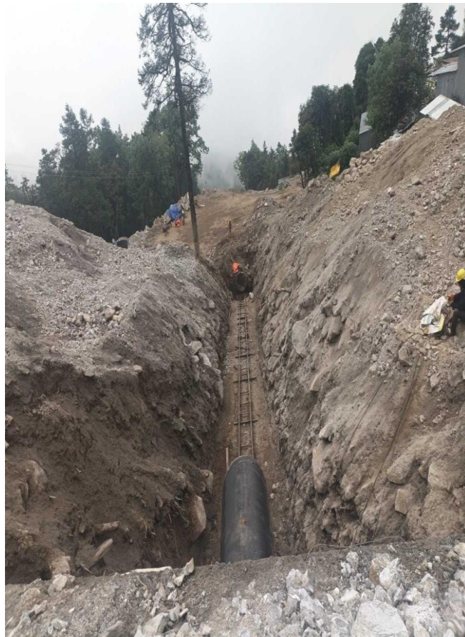
Concreting at AB-1 d/s at Penstock Alignment.
