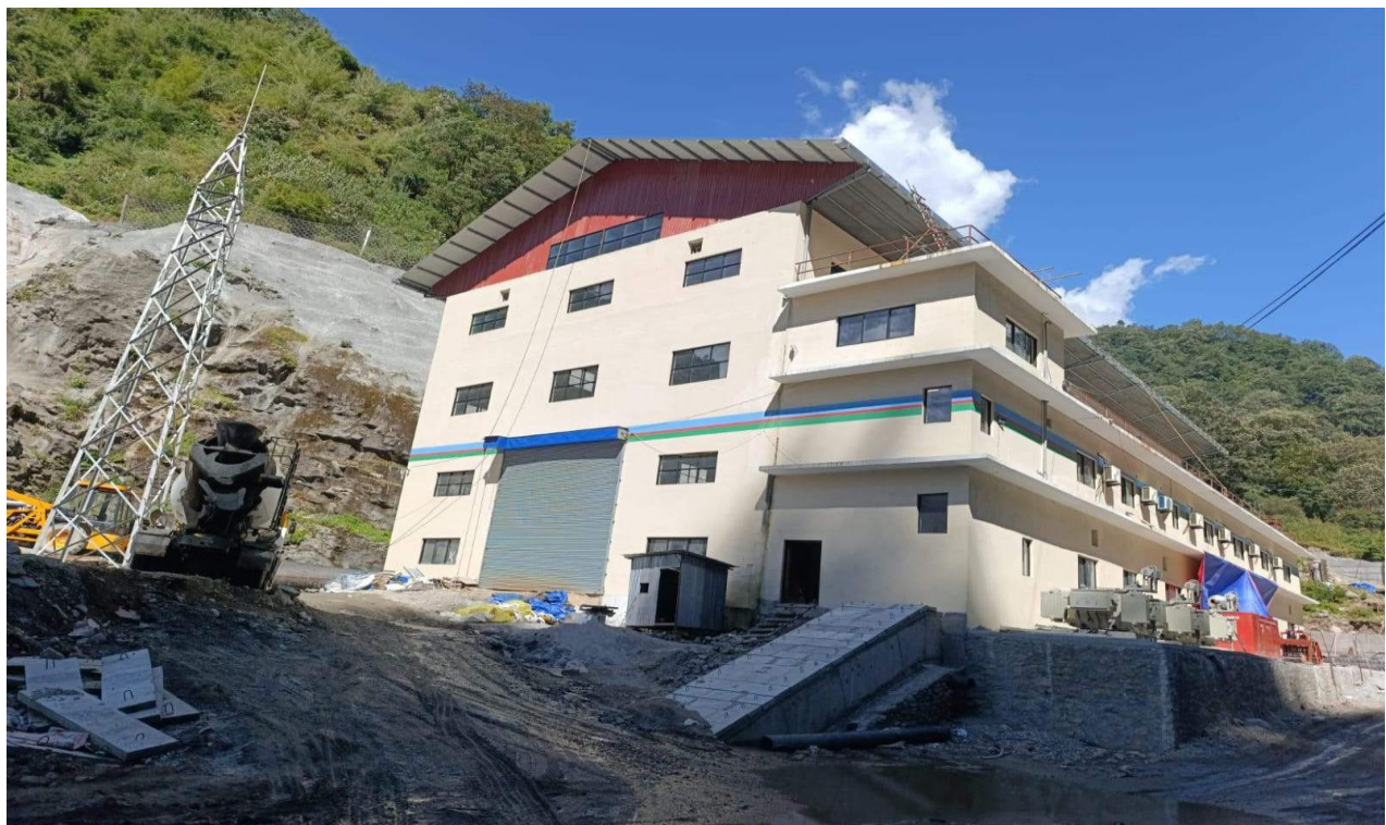
Powerhouse and Control Building
