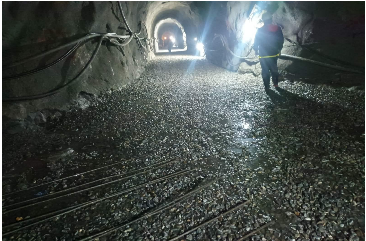
Base Preparation for Invert Concreting
