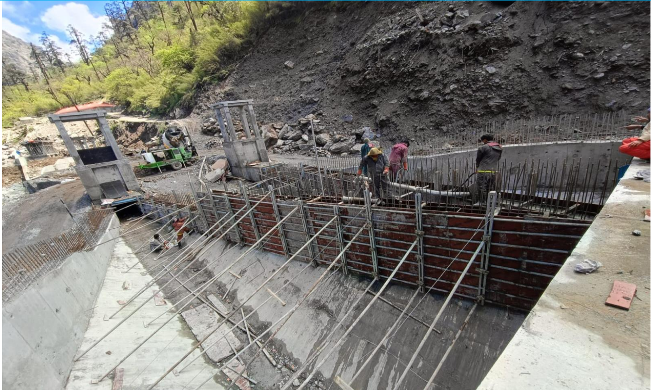
Concreting at Settling Basin
