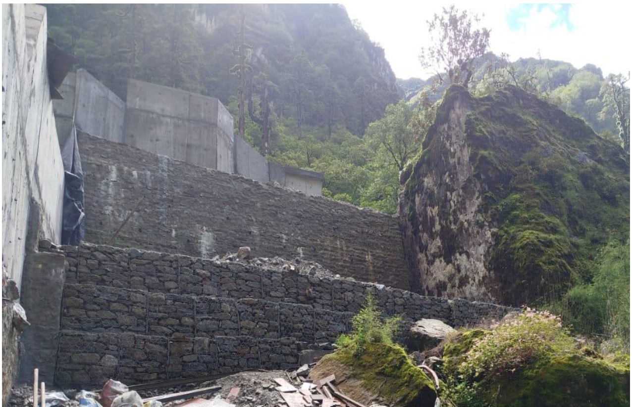
Nupche Headworks Spillway
