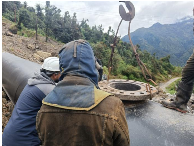
Manhole installation
