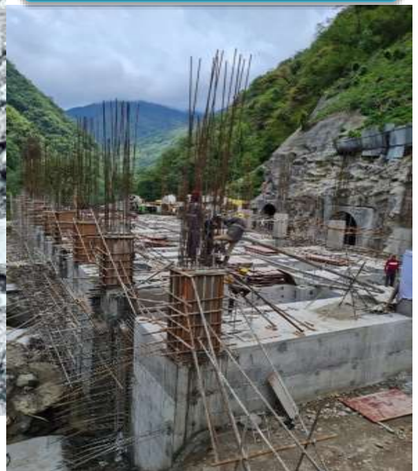
Erection of Powerhouse Column
