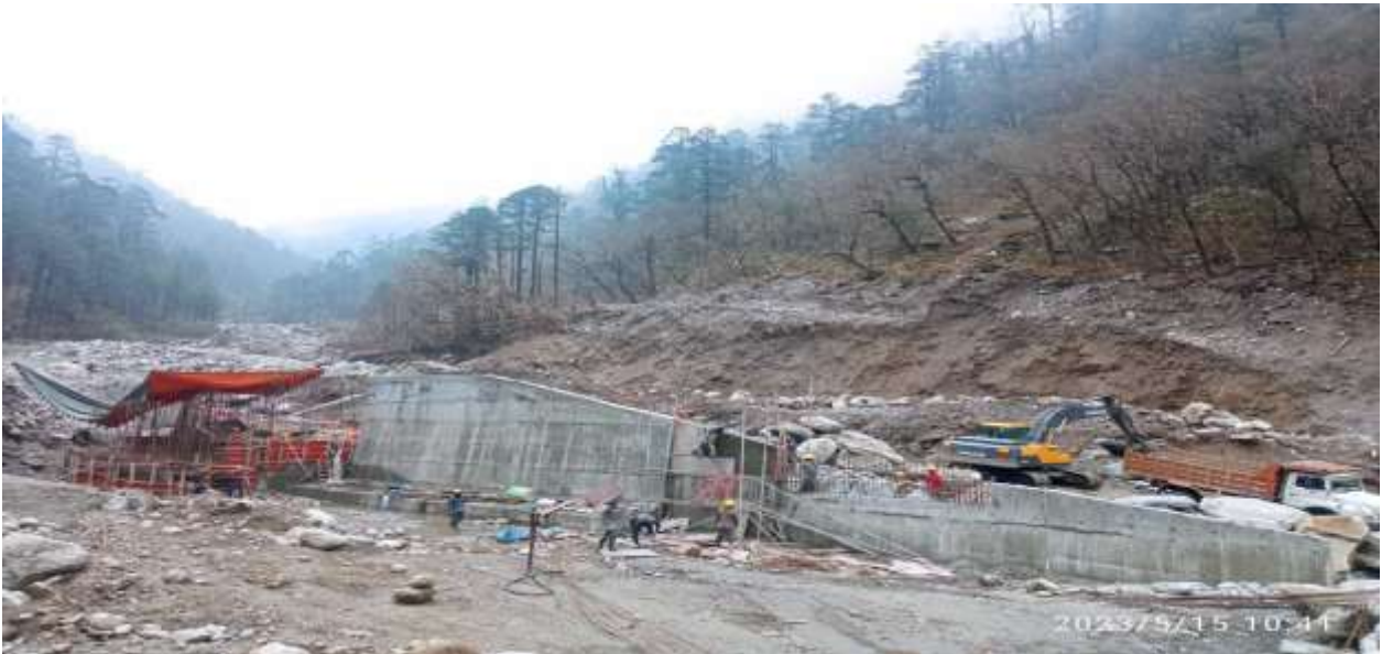
Likhu Headworks Components; Headworks, Settling Basin, Flood Wall
