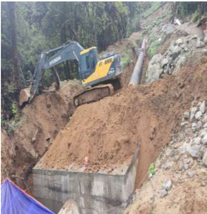
Backfilling of Anchor Blocks
