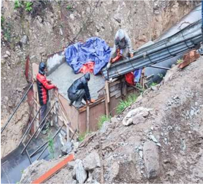
Concreting of Anchor Blocks
