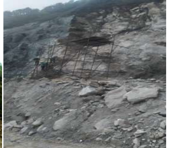
Additional Support in Surge Shaft
