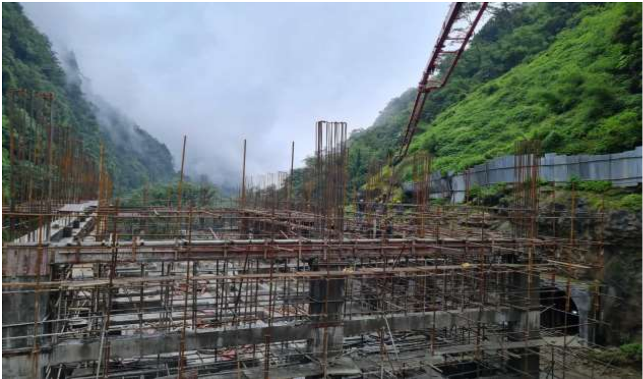
Progress in Powerhouse
