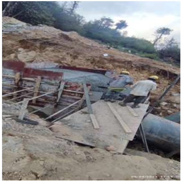
Concreting of Anchor Blocks
