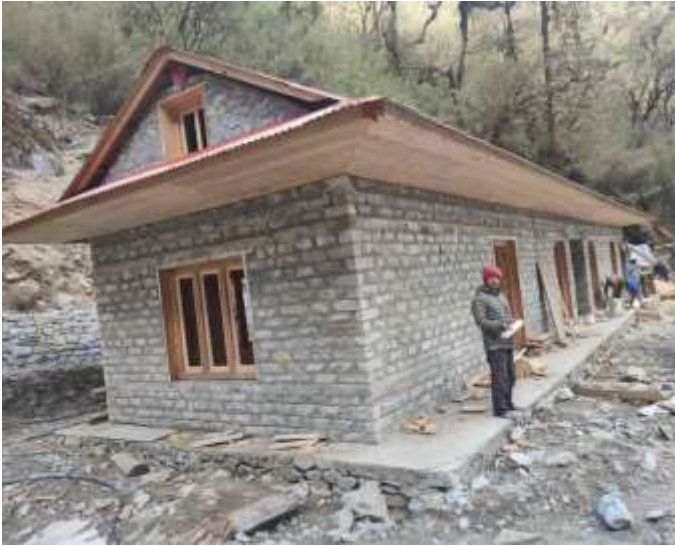
Execution Infrastructures in Construction Site
