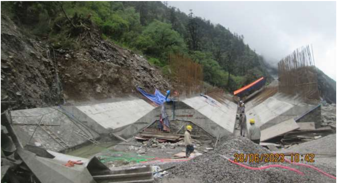
Nupche Settling Basin
