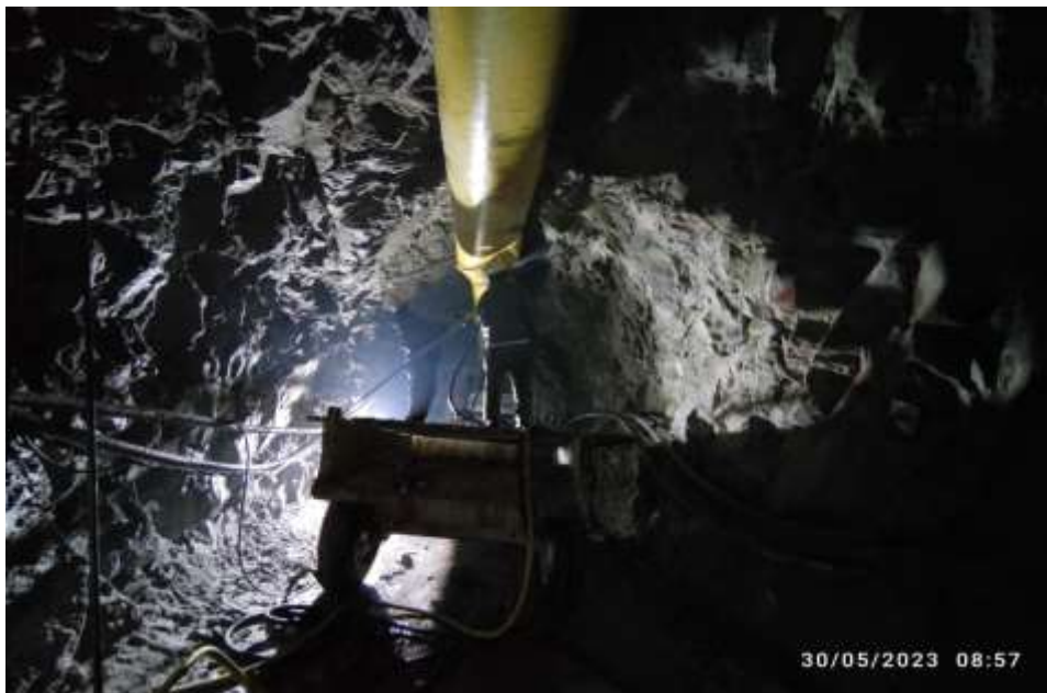
Tunnel Excavation Process and Support Works
