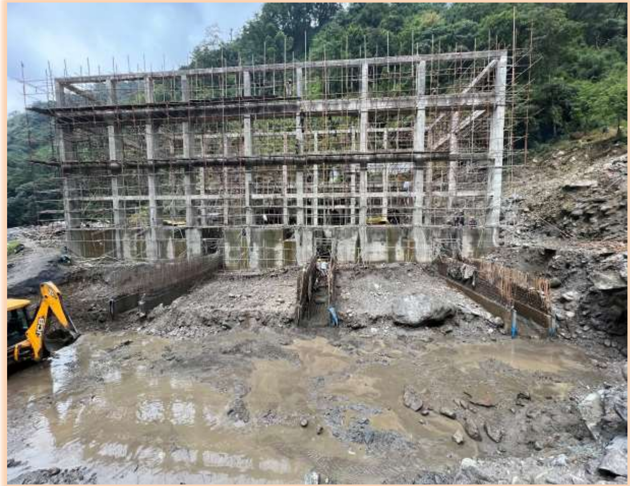
Excavation of Tailrace Works
