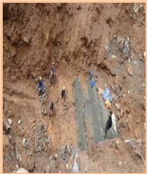
Masonry works at Penstock
