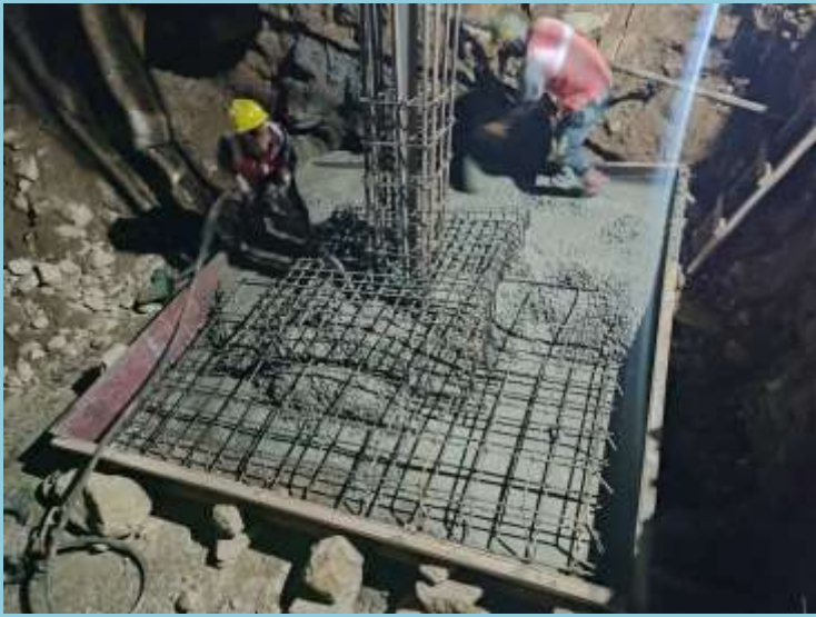
Concreting at Foundation pit.
