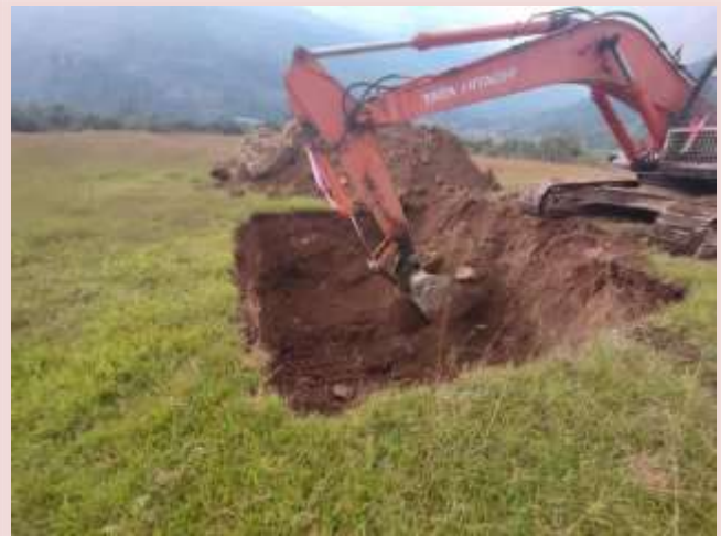
Foundation pit marking of Transmission line(Left) Excavation of foundation(right)
