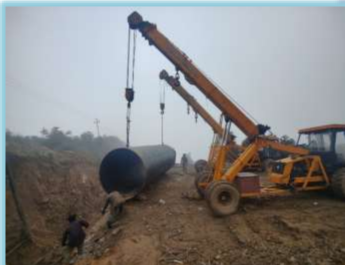
Lowering of pipes
