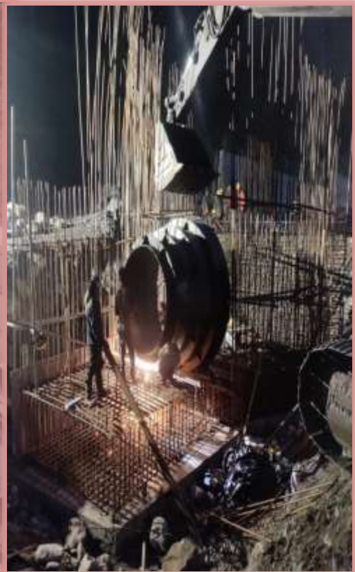
Erection of Bell mouth at Likhu HW
