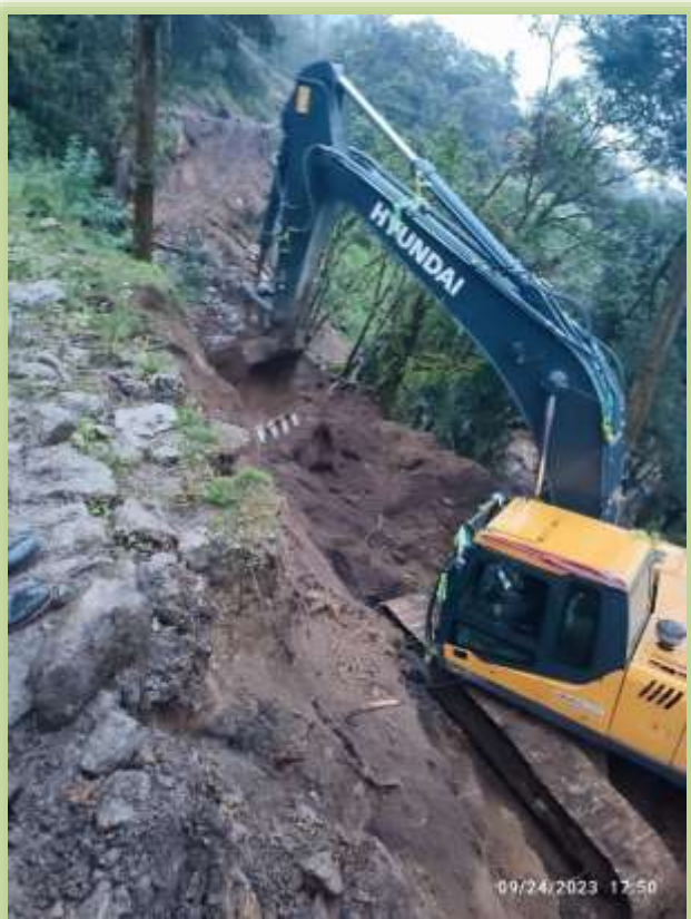
Road Diversion at Penstock
