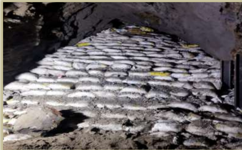
Cavity protection at Likhu Inlet; Chainage 1+029
