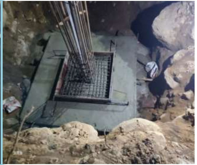
Concreting at Foundation pit.
