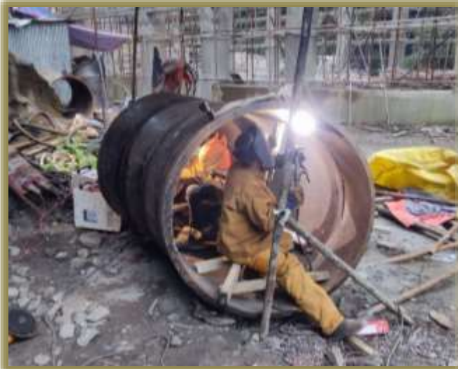
Fabrication of VS2 Bend
