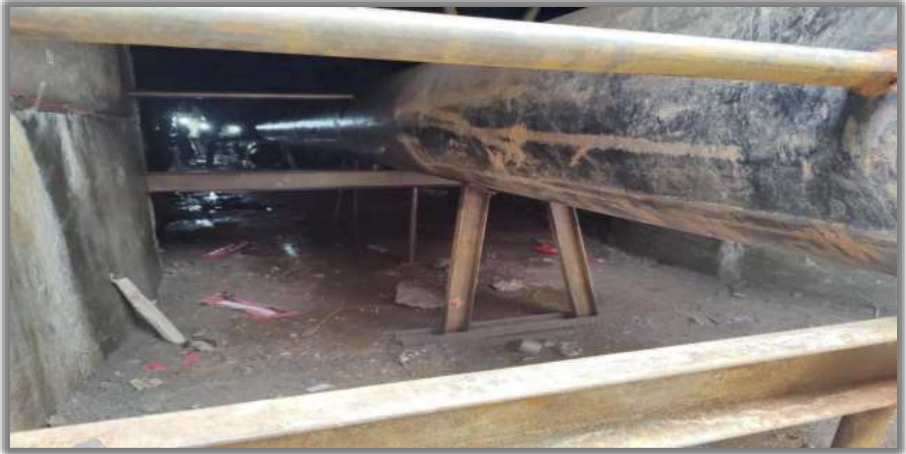
Branch pipe installation with saddle support
