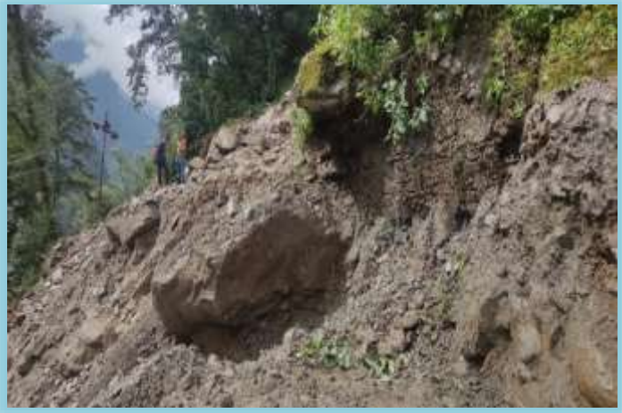
Access Road Blockage
