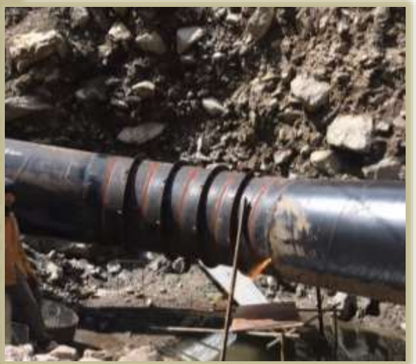
Erection of Bend 12 at penstock
