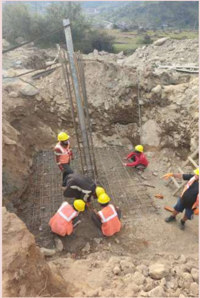
Field Density Test for Foundation of Transmission line(Left) Placement of rebar in foundation(right)
