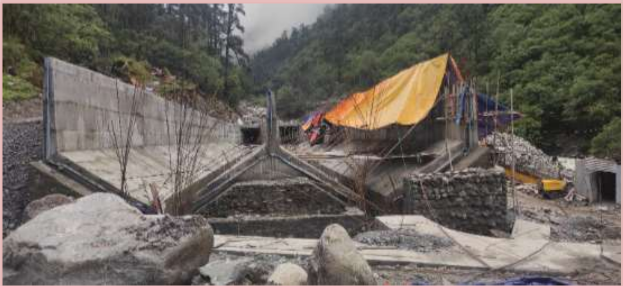
Nupche Settling Basin
