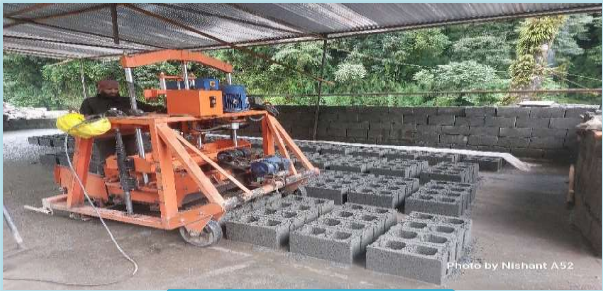
Block Production for Exterior wall
