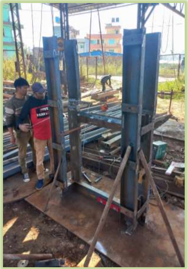
Fabrication of Frames for gates in workshop
