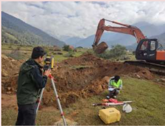
Foundation pit marking of Transmission line(Left) Excavation of foundation(right)
