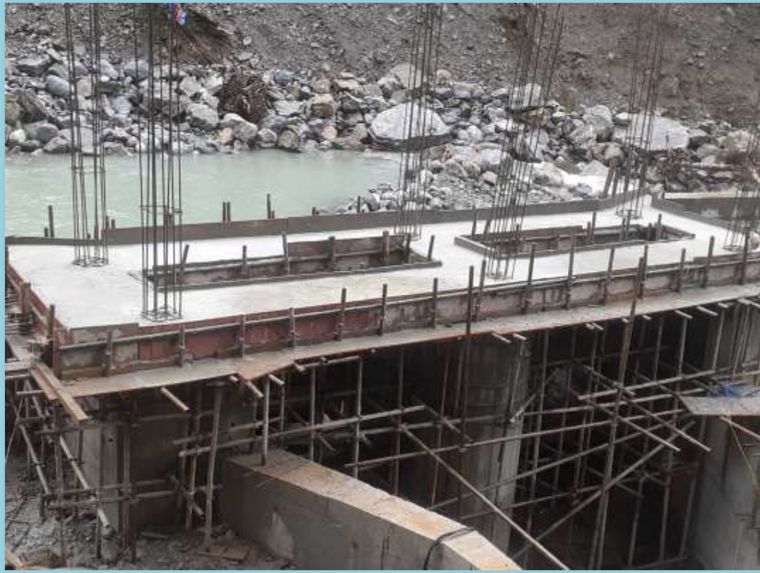
Likhu Intake Top slab
