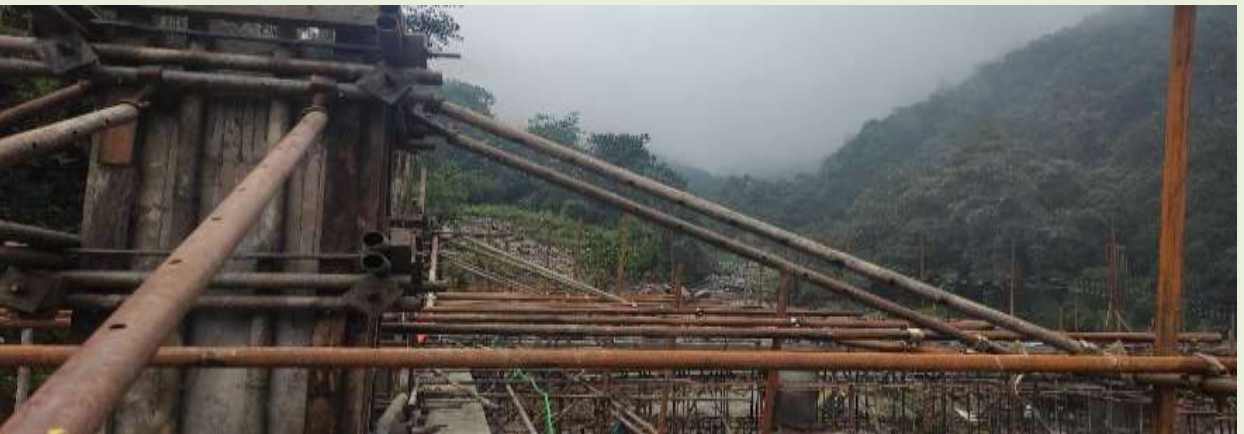
Erection of Powerhouse Column
