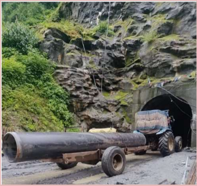
Pipe Transportation at Nupche yard
