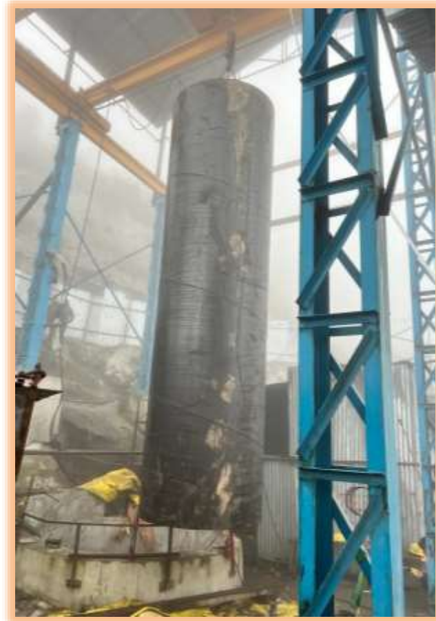
Loading test of Pipes at vertical shaft
