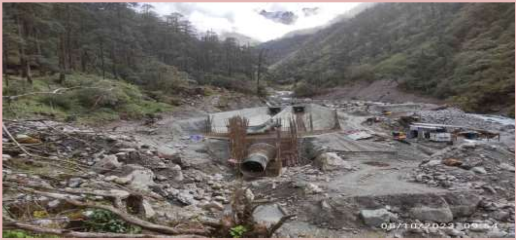
Gravel Trap at Likhu Headworks
