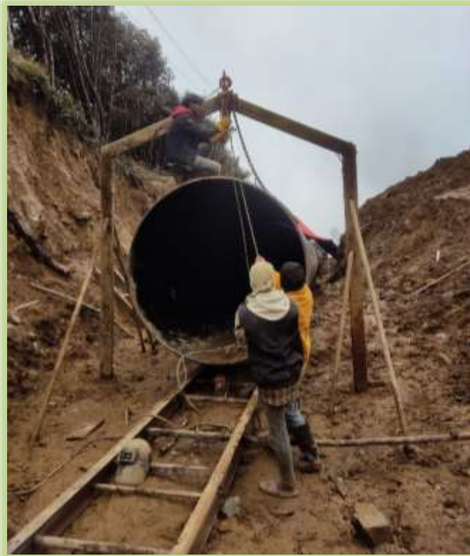
Fitting of Pipes at Likhu HRP
