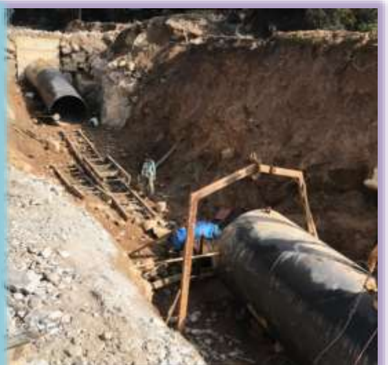
Fitting of pipes
