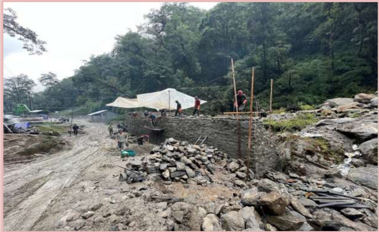
Masonry works at Boundary at Switchyard protection
