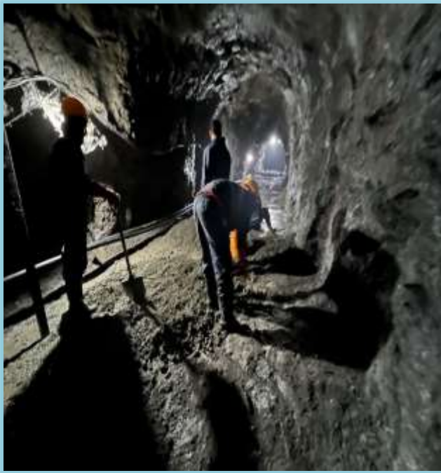
PCC at inclined Tunnel
