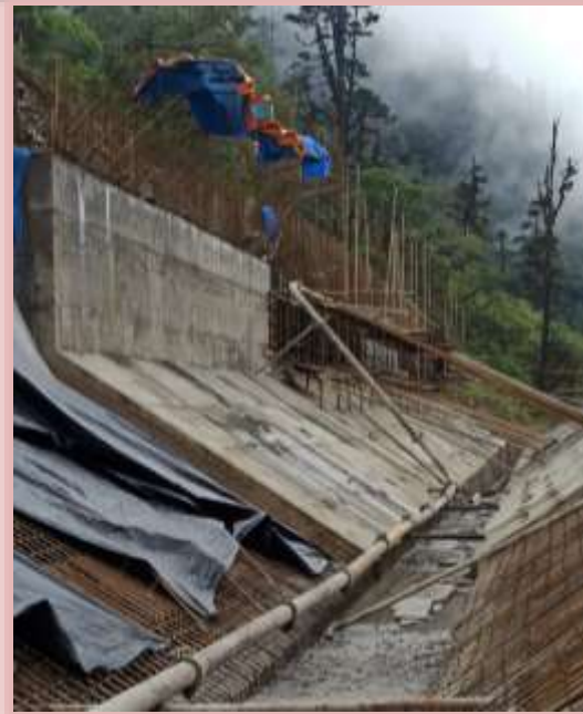
Nupche Settling Basin
